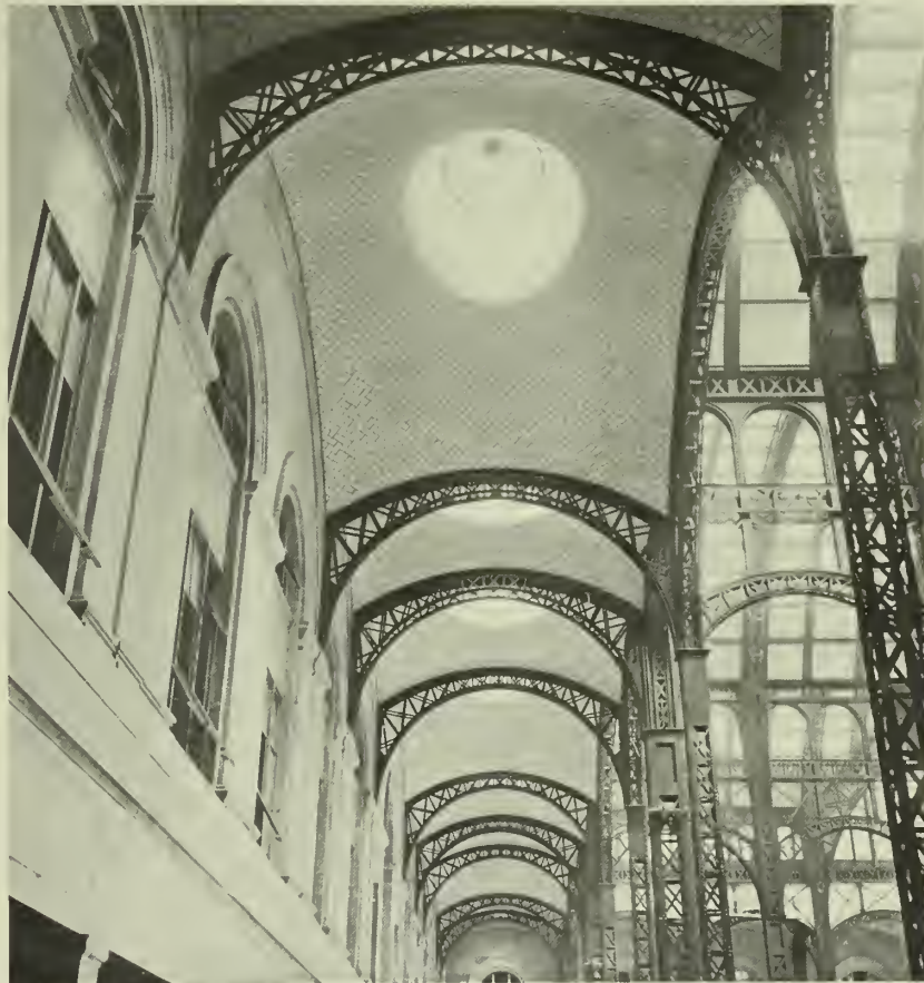
CONCOURSE OF PENNSYLVANIA RAILWAY STATION, NEW YORK CITY. Vaulted ceiling of Guastavino construction. McKim, Mead & White, Architects.
